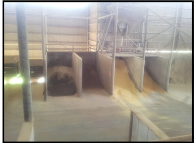
Storage bins at CPC Commodities.
